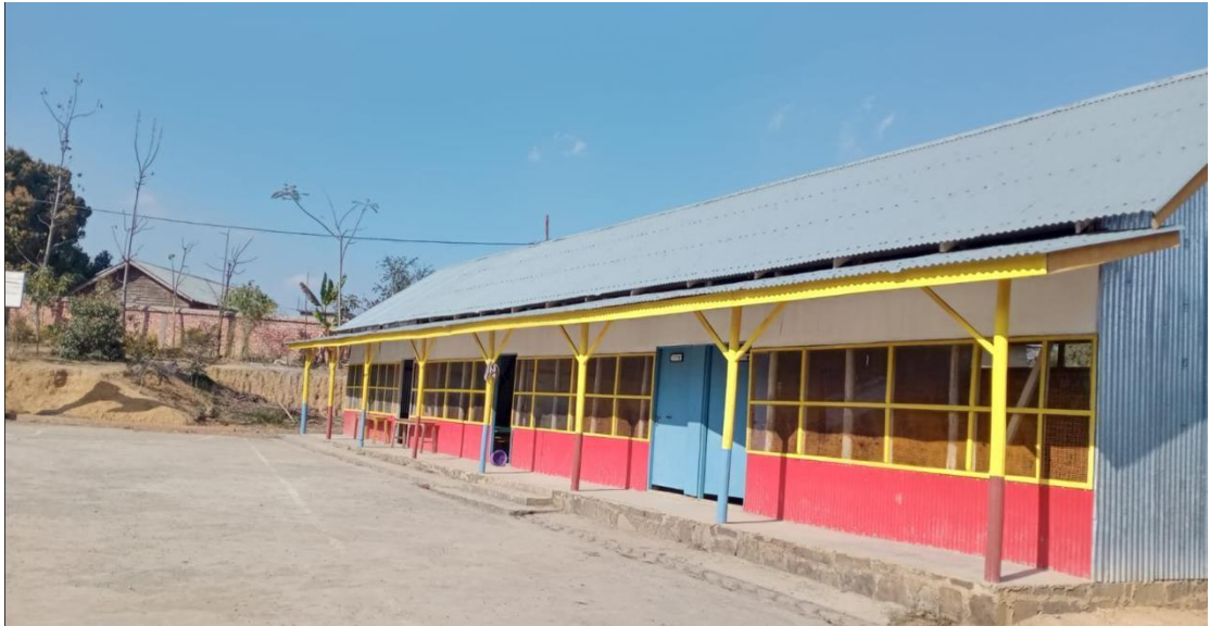
Figure 4. 5: Kindergarten Block of Gateway School
