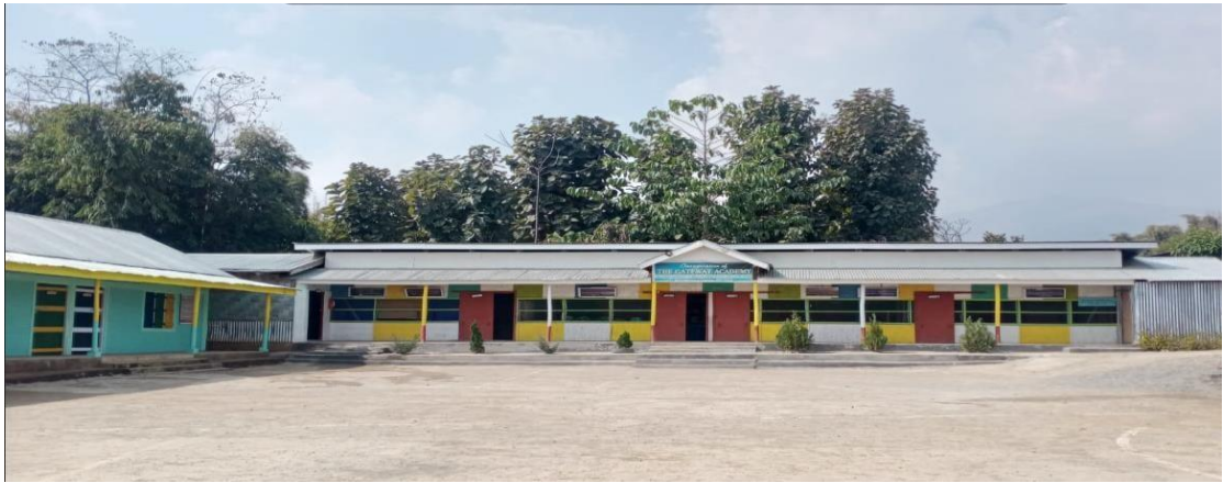
Figure 4. 4: Main Building of Gateway School
